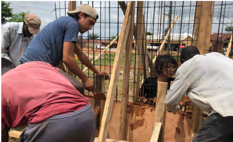
Construction site -- pouring red-earth wall mixture [Image 11]
