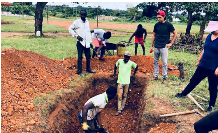
Construction site -- digging. [Image 6]
